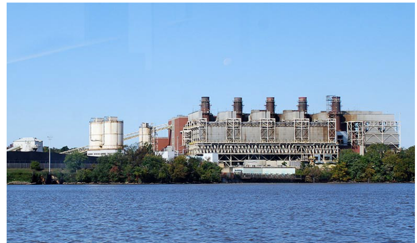
Old Town North - Existing Power Plant Structure
