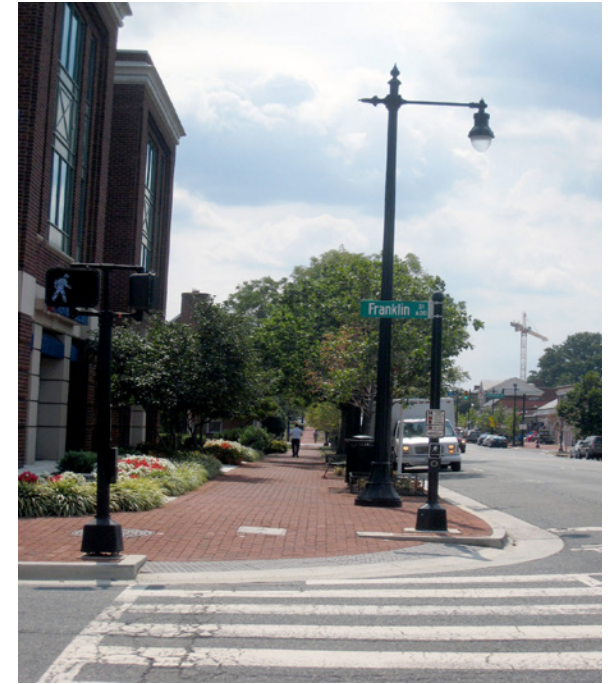
Streetscape improvements on S Washington Street, utilizing the light fixture (GWMP Parkway Streetlight), pedestrian curb ramps, rationalized furniture placement and brick paving which are required in these Design Standards and Guidelines
