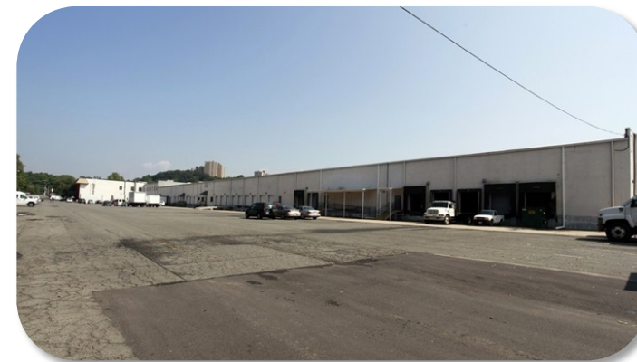
Figure 53: Plaza 500, 6259 Edsall Road Source: CoStar
