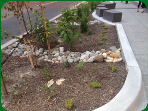
Bioretention, 19th ST NW, Washington DC
